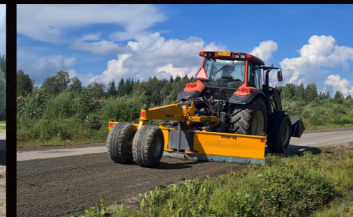
MGR-420 Gravel road maintenance
