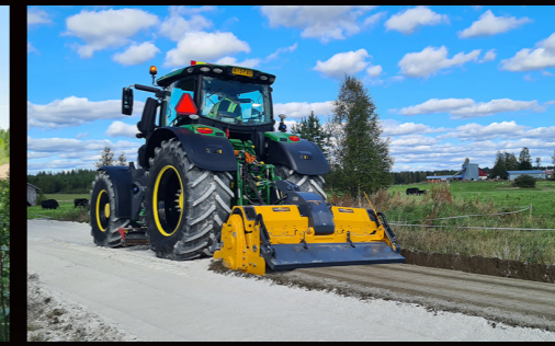
RC65 Stabilization and mixing of binders
