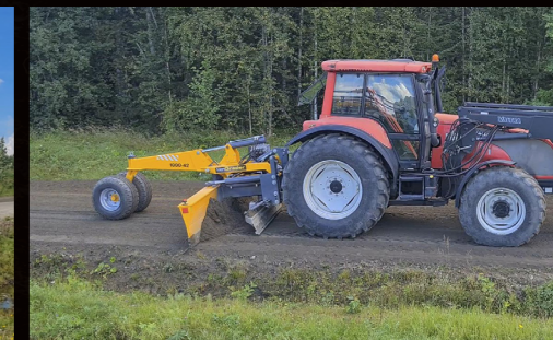
MGR-420 Gravel road maintenance
