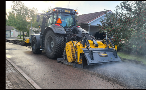
RC90 On-site asphalt recycling
