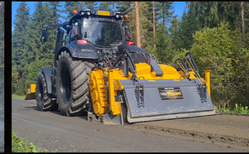
RC90 Gravel road maintenance
