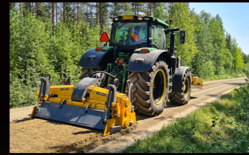
RC65 Gravel road maintenance
