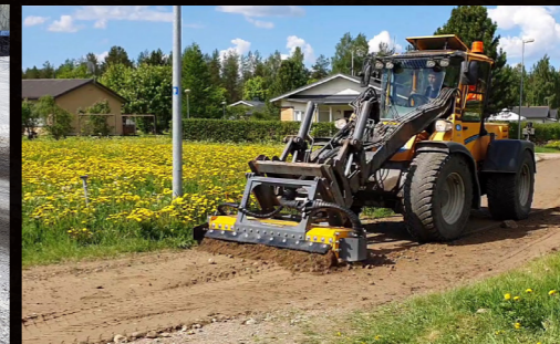
MC4 Gravel path maintenance
